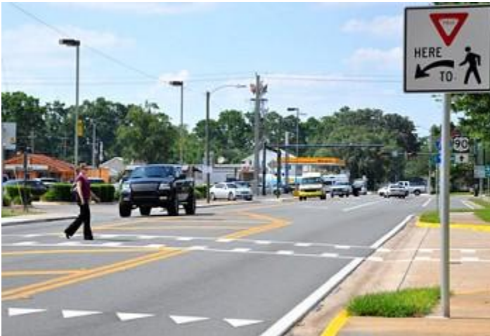
Squares in the crosswalk mark the safe area for pedestrians and 'shark's teeth' show where vehicles must stop at this new crosswalk on S. Marion Avenue. (FDOT photo)
